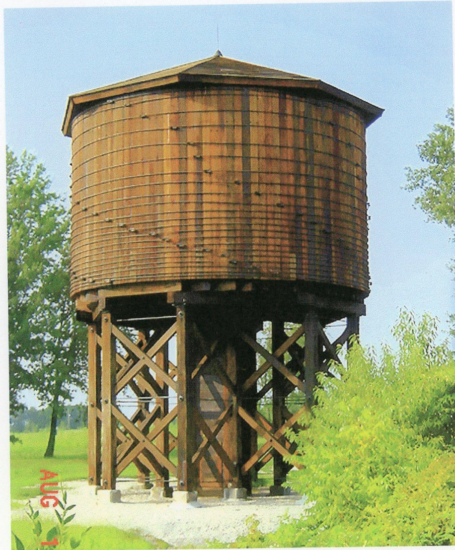
RESTORATION OF THE ILLINOIS CENTRAL RAILROAD WOOD WATER TANK AND TOWER, CITY OF KINMUNDY, ILLINOIS
