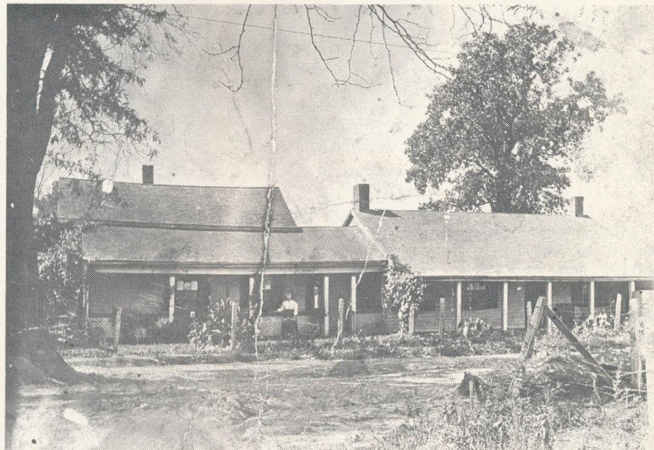
THE ORIGINAL Castle home on West Whittaker street facing South Castle street, Mrs. Belle Castle is standing in front of her home. This home at this time was one of the show places of Salem. It burned about 1920. They
