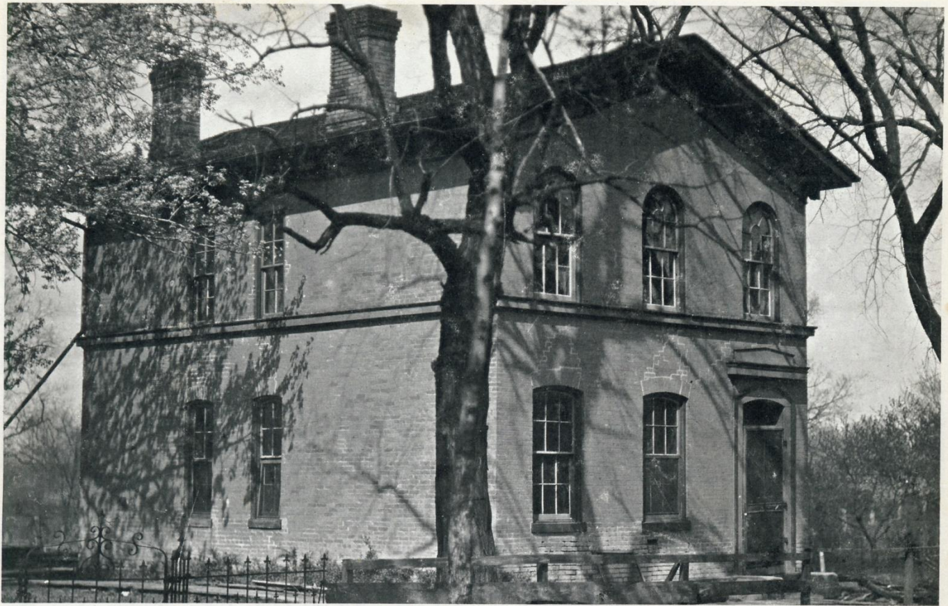
The Marion County Jail: The third jail built in December of 1854. It was the first county building to be built of brick. The jail was located in the same block as the present jail. The jail was built at a cost of $3,937.00. The first two jails were made of logs. The first jail was an unheated, unlighted log structure with a cell in the interior. The cell resembled a huge box which had a trap door in the top by which the prisoner was lowered in from the ceiling.
