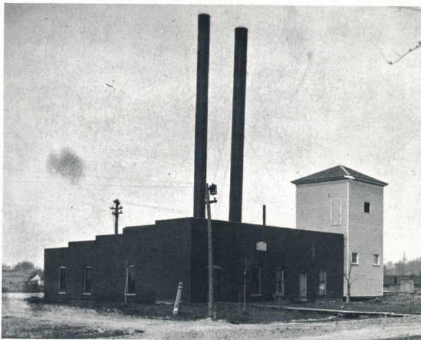
Electric light plant, Salem, Ill. Constructed in 1898.
