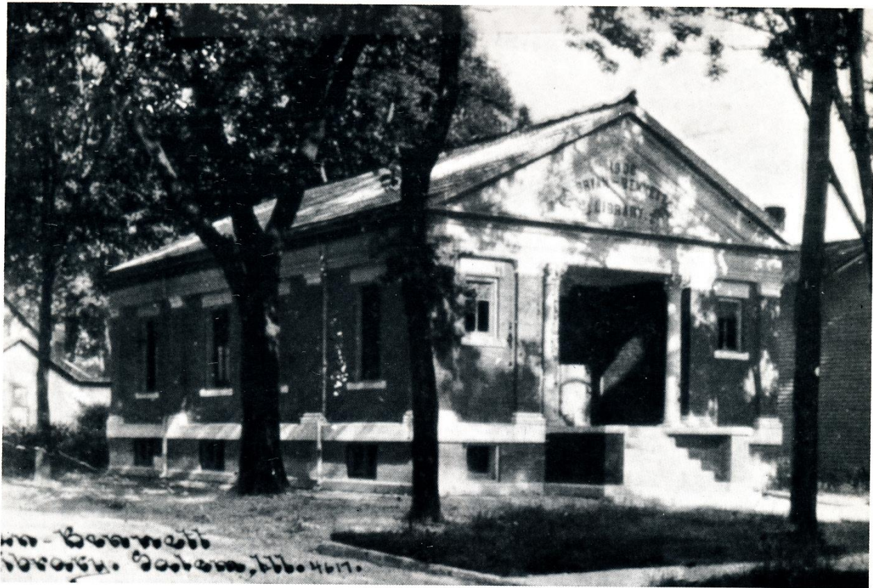
Bryan Bennett Library constructed 1908.
