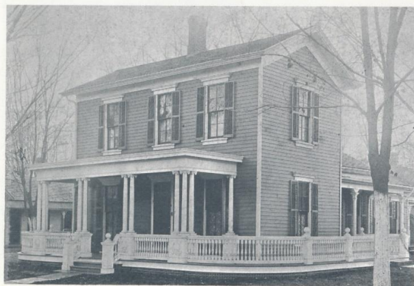
The home of Frank Bradford, located at the southwest corner of Washington and McMackin, 1903.
