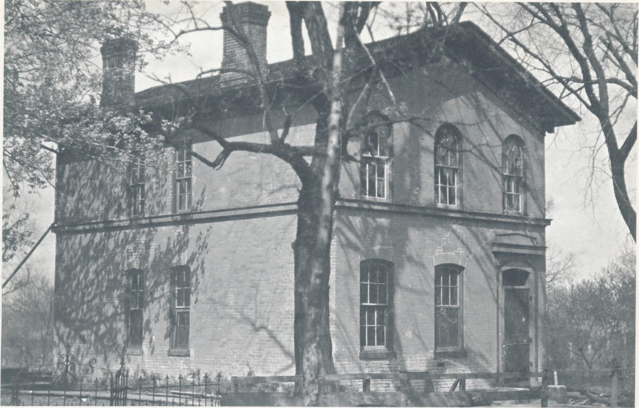
The Marion County Jail: The third jail built in December of 1854. It was the first county building to be built of brick. The jail was located in the same block as the present jail. The jail was built at a cost of $3,937.00. The first two jails were made of logs. The first jail was an unheated, unlighted log structure with a cell in the interior. The cell resembled a huge box which had a trap door in the top by which the prisoner was lowered in from the ceiling.
