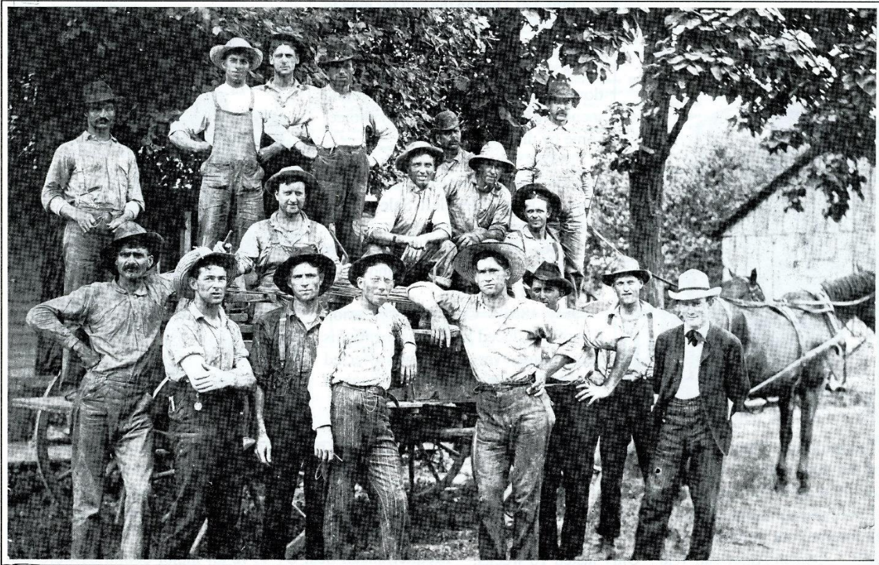
This telephone line crew was hired at a rate of 10 to 20 cents per man per hour in about 1905.
